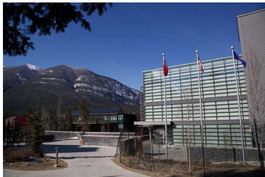
The Kinear Centre for Creativity & Innovation at the Banff Centre hosted the 2015 Banff Pipeline Workshop.
